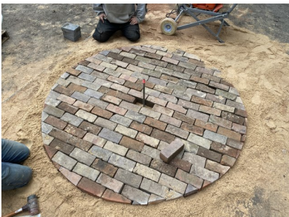
The labyrinth in progress
