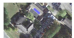
Solar panels on two FPCOR buildings
