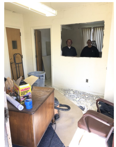
Dan Blandford and Joe Everitt take a pause from renovation work.
